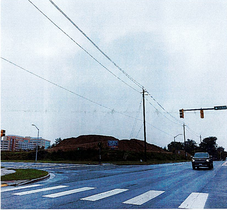
Figure 6: Site view from Cherry Hill Road.
