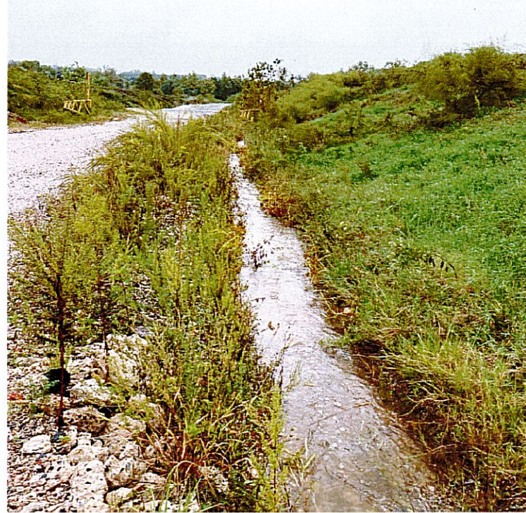
Figure 7: Haul road, berms, and drainage.
